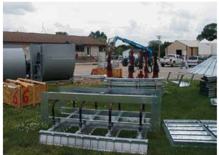
At StateLine Cooperative's Ringsted location, a new continuous flow natural gas dryer is being built to provide increased drying capacity system-wide.
